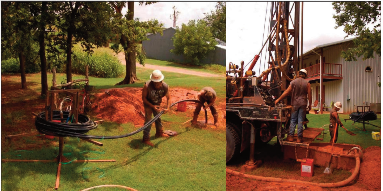
FIGURE 4. Underground loop installation at participating home. Source: www.wfec.com/portal/marketing/communications/photo-galleries/geo-drilling
