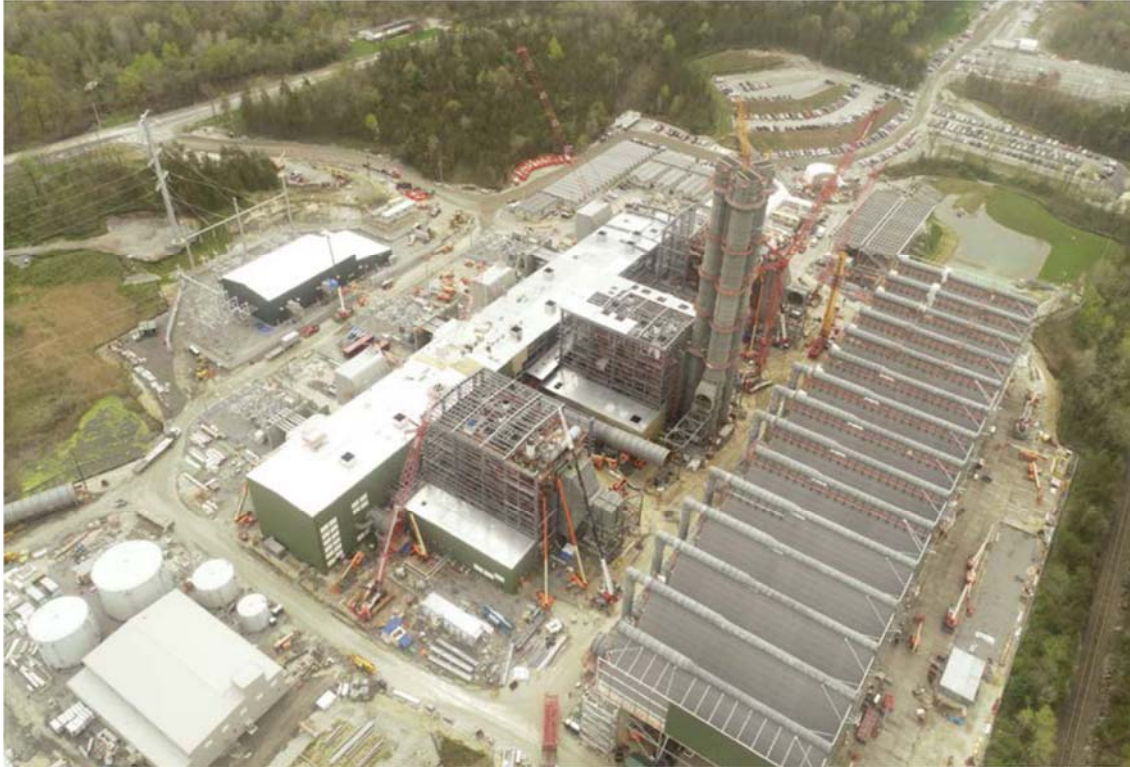
Construction Progress, Looking Southeast
