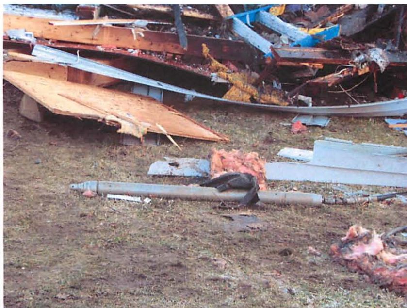
Image #2 – Pneumatic Bullet Used by Contractor – Taken by Arpit Mehta
