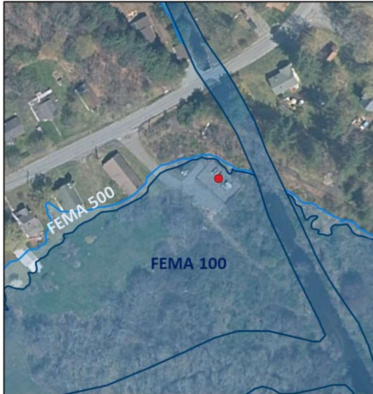
Figure 2. Summitville Substation yard (red dot) is located next to the Delaware and Hudson Canal and is within the FEMA 100-year flood plain extent
