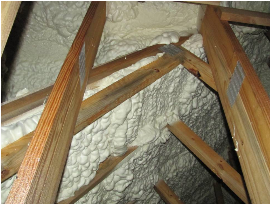
Figure 2: Photo of Roof Insulation
