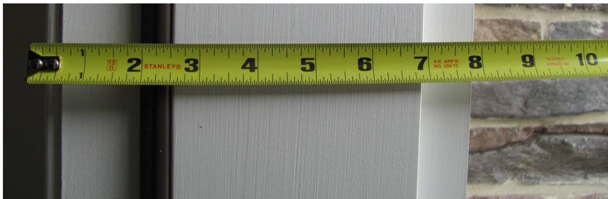
Figure 1: Photo of Wall Thickness
