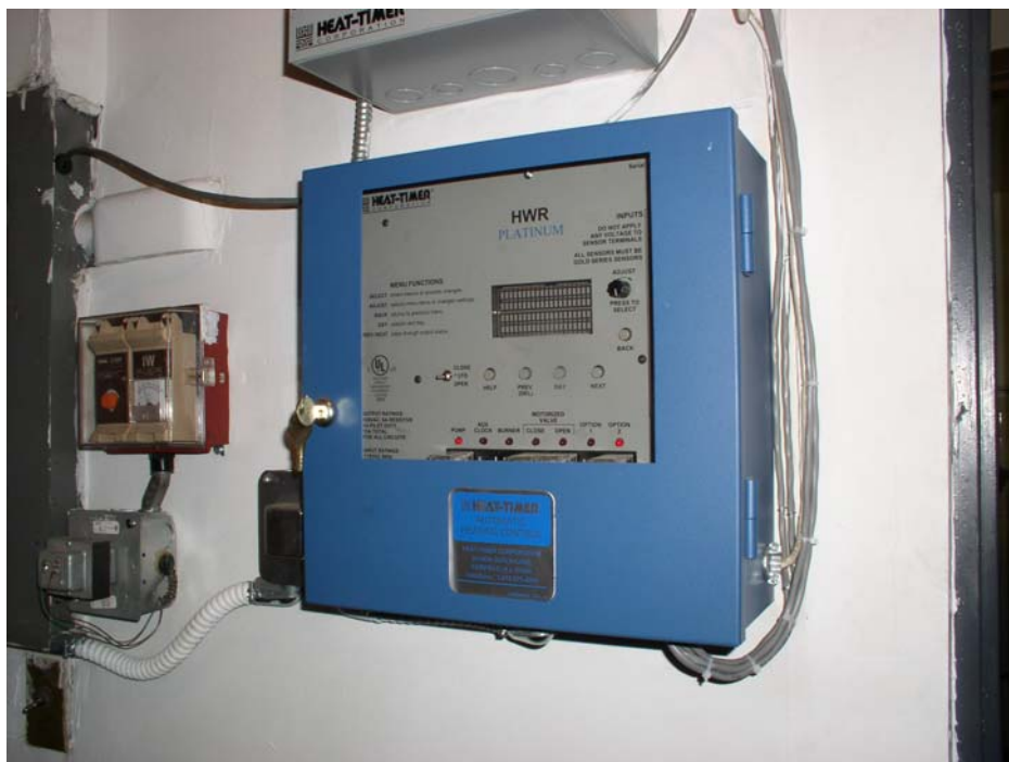
Figure 1: Heat-Timer HWR Platinum Controls
