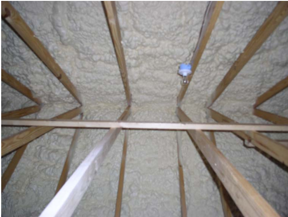
Figure 1: Photo of Roof Insulation
