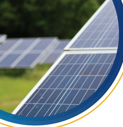
Additionally, the solar panels are mounted at an angle that allows for the most light to be absorbed throughout the year, which results in the panels facing the sky at shallow angles (typically less than 25 degrees). As a result, what little light is reflected is not visible to ground-level observers.
