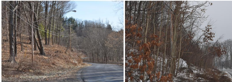
Figure 1. Left: Maintained right-of-way, light brush. Right: Without herbicides brush grows into small trees
