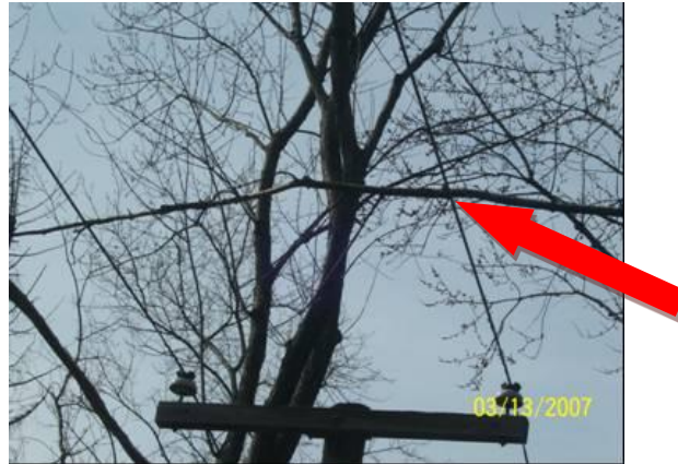
Figure 10. Small, dead, silver maple branch across two phases spaced relatively far apart (low voltage gradient) did not result in an interruption
