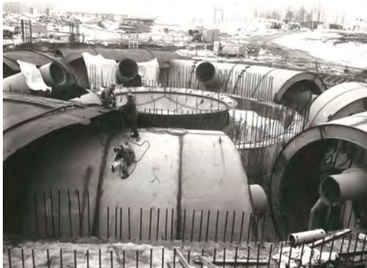
1969 construction photo - building FitzPatrick's Torus
