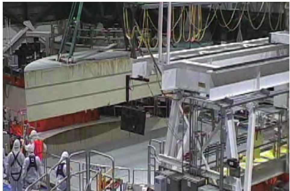
The “all rods in” announcement this morning was the cue for the Refuel Team to start reactor disassembly. The picture above was captured shortly after the announcement.
