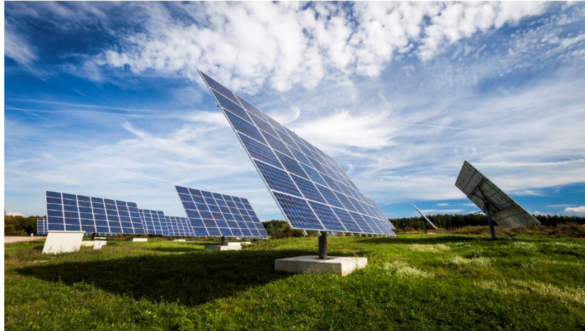
Photo 18: Dual Axis Panel Installation (Photo Credit: Deger energie Gmbh & Co. website)
