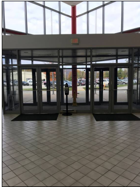
Figure 10 Views of Subject Office Building Lobby
