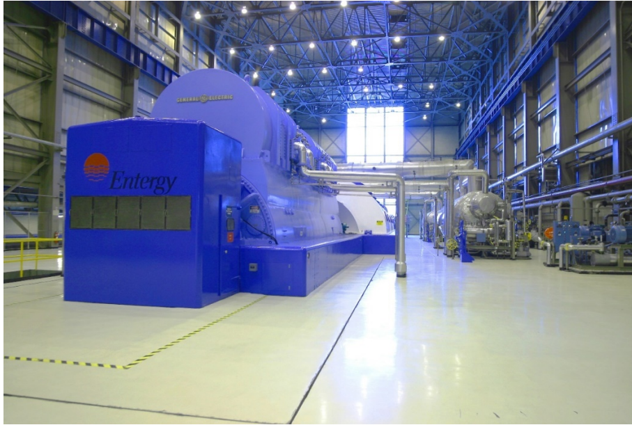
Photo 4: Indian Point Unit 2 Turbine Building
