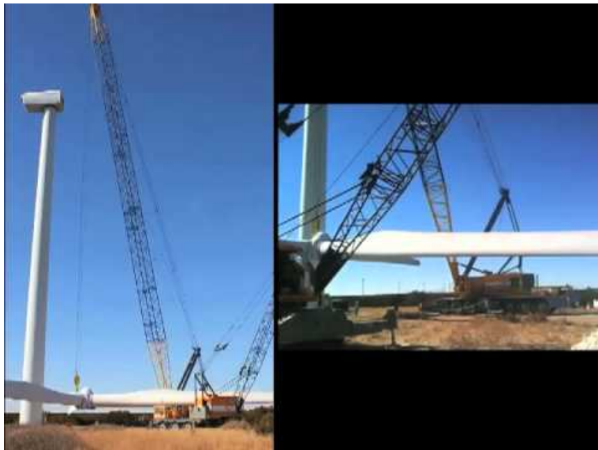
Photo 15: Turbine Rotor Lift
