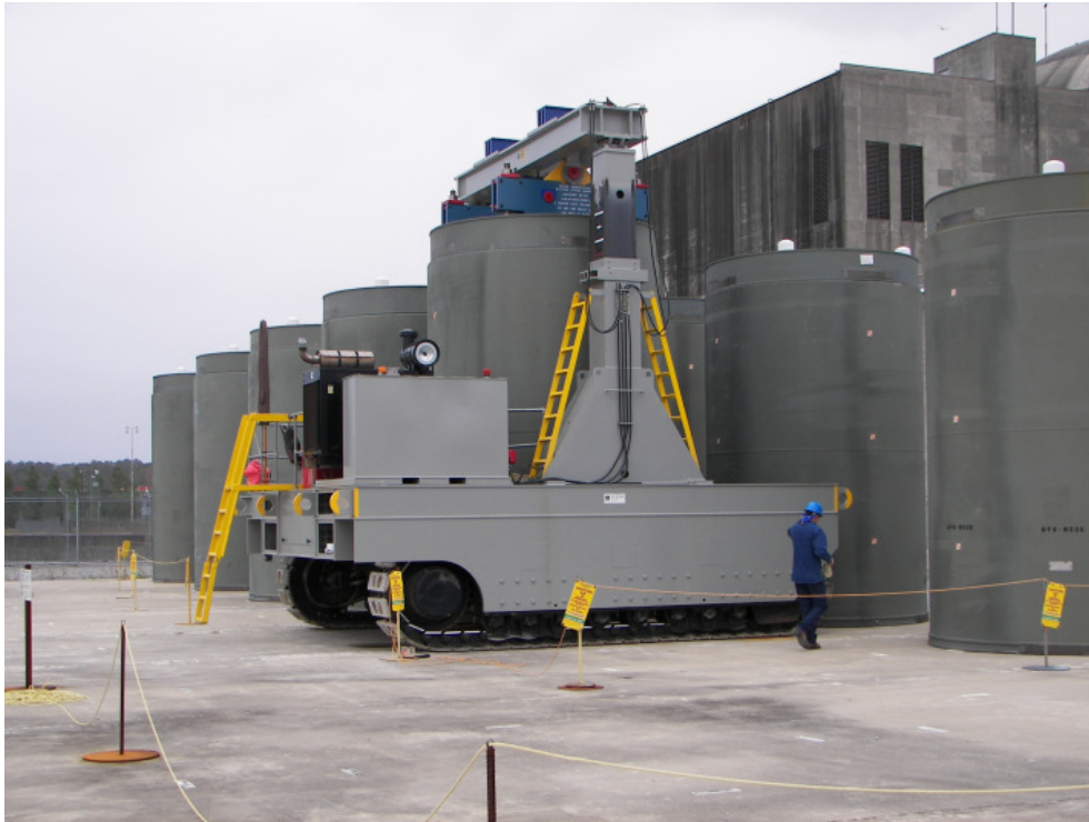
Photo 7: Holtec Inc. HISTORM Dry Casks and Transfer Device
