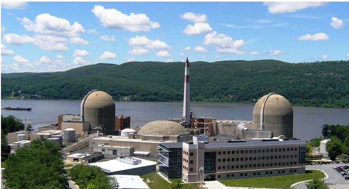
Photo 1: Indian Point Energy Center - Units 1, 2, and 3
