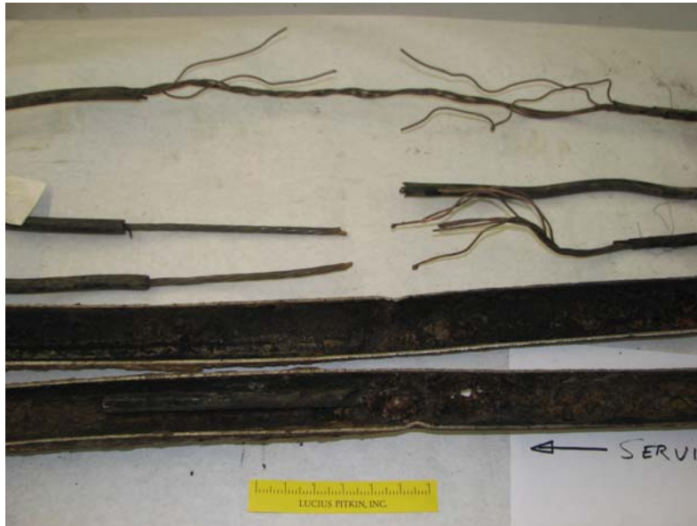
Photo 4 - Electric conduit and cables 19 feet from gas main crossing
