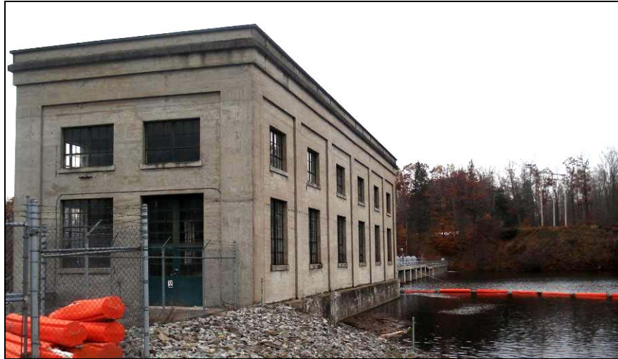
Photo II-8 Brookfield's Generating Station at the Lighthouse Hill Site
