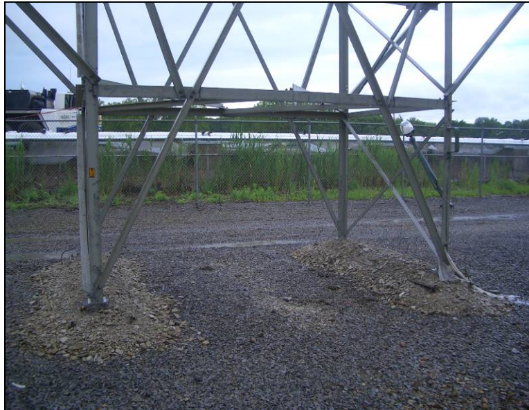
Photo II-4 230kV Structure Foundation at Dunkirk
