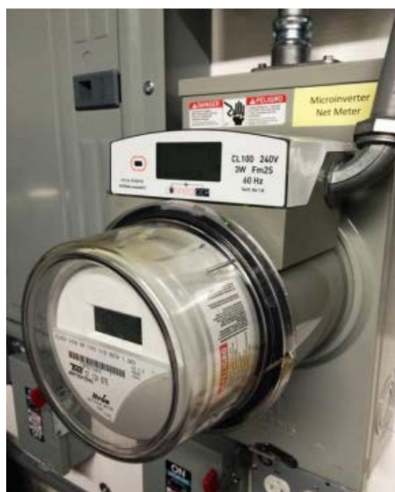
Figure 19: ConnectDER™ Meter Collar
