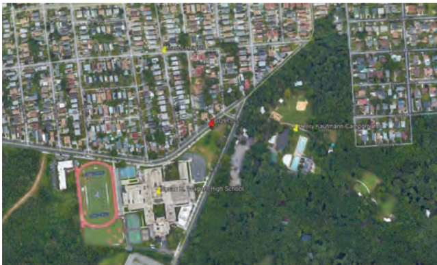
National Grid | Governor 305 Regulator Station | December 2019
