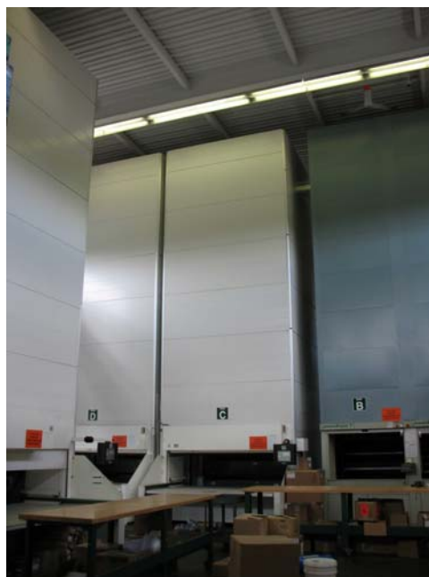
Figure 27: BCW Storage Towers 1001
