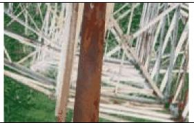
Rating 4 - "Light Pitting" Some very light edge roughening. Loss of greater majority of coating and zinc layers. Corroded surface would dominate surface preparation - remedial action using wire brush, scraper and brushed paint not sufficient to give greatly increase life
