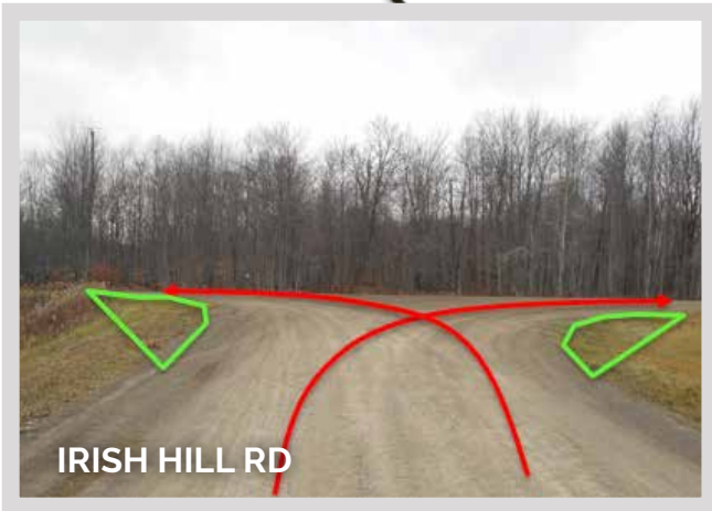
Intersection of Irish Hill Rd and Keenan Rd measured 110ft, both northeast and southeast areas need to be modified
