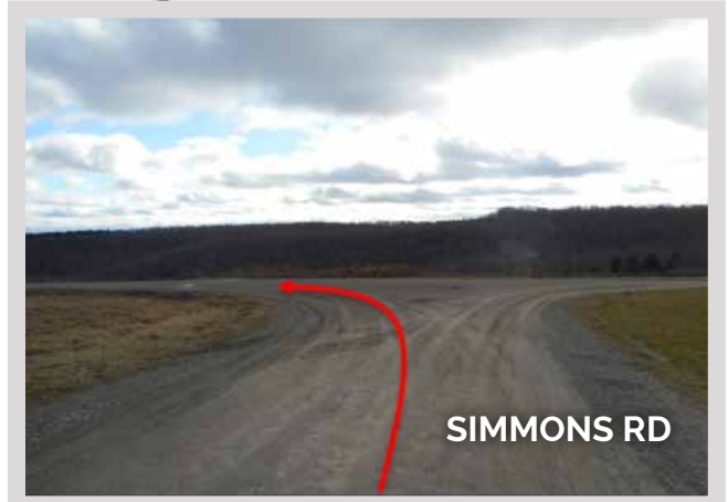
Intersection of Simmons Road and Dryden Hill Road measured 95ft, northeast corner needs to be modified.
