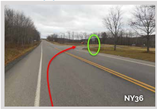
Intersection of NY36 and NY417 in Jasper, measured 130feet. Turn was slightly short and need signage removed in north corner.
