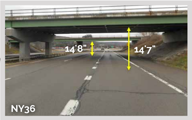
NY36 under Int86, measured 14'7 at the lowest
