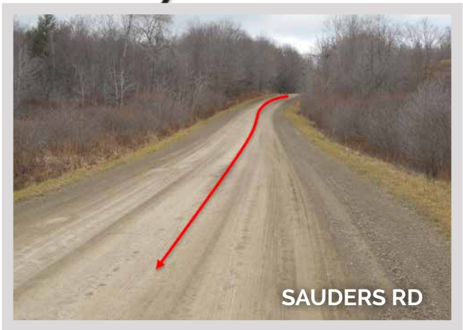
Sauders Road, windy road with some trees which will need to be trimmed.
