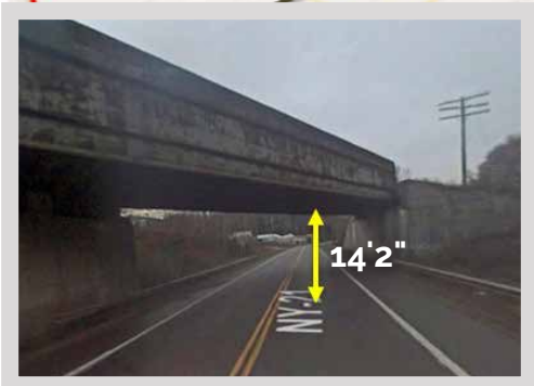
NY21 rail overpass in Alfred Station
