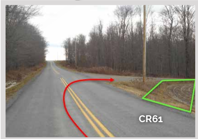
Intersection of CR61 and Pease Rd measured 100ft, Logisticus recommends a cut through to avoid the utility pole.
