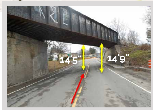
NY417 train overpass in Wellsville
