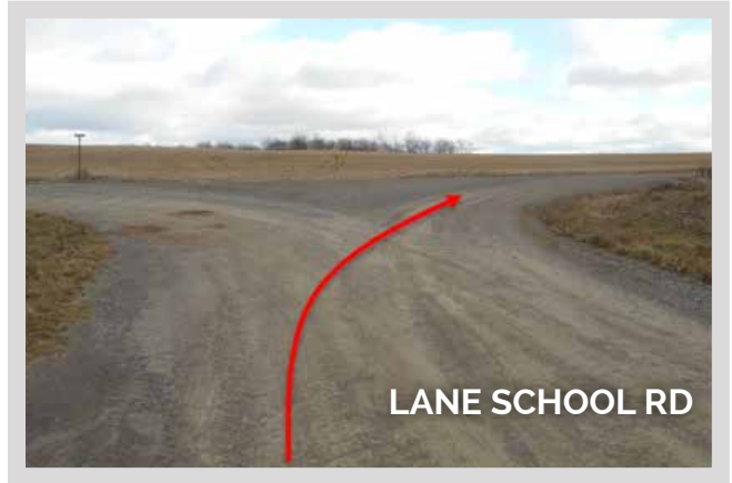
Intersection of Lane School Road and Simmons Road measured 120ft, southwest corner needs to be modified.
