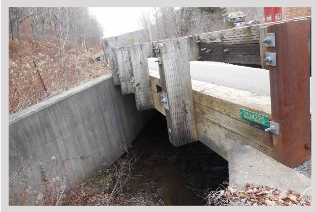
Bridge 1 of 3 on County Road 98 – Tiber Deck
