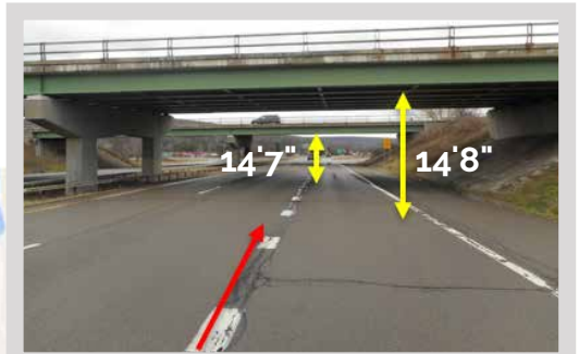
Hwy36 underpass under Int86 in Hornell
