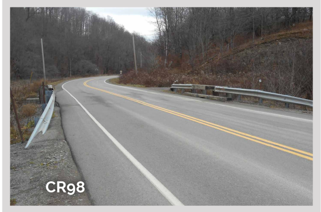
Bridge 1 of 3 on County Road 98 – needs 3rd party review
