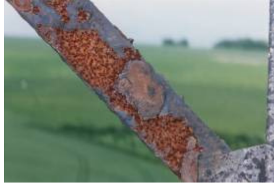
Visual Rating 5 – Significant Pitting Significant pitting – loss of section clearly visible, edges feathered/thinned
