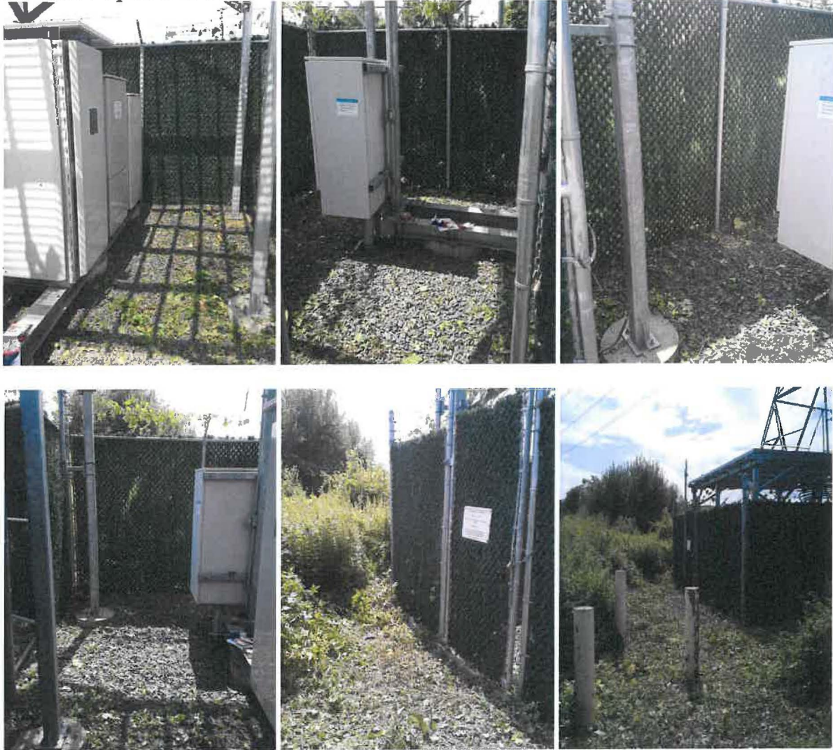
Site Clean-Up Post-Work:
