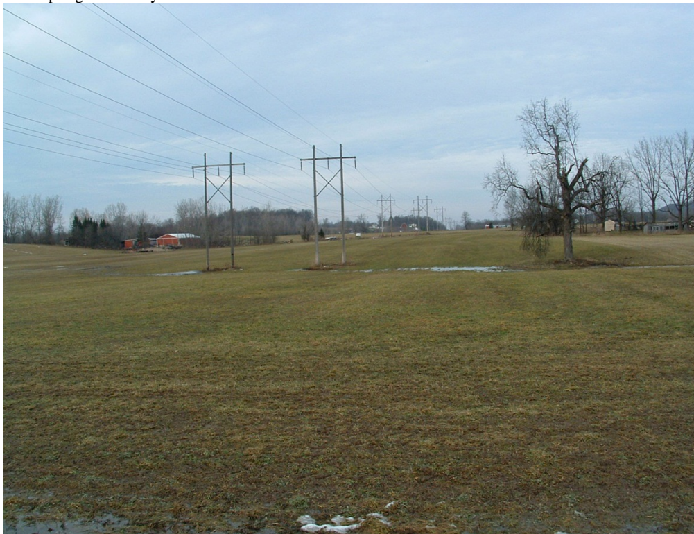
Figure 4-6 Existing NYSEG ROW looking north at Reyer Road
