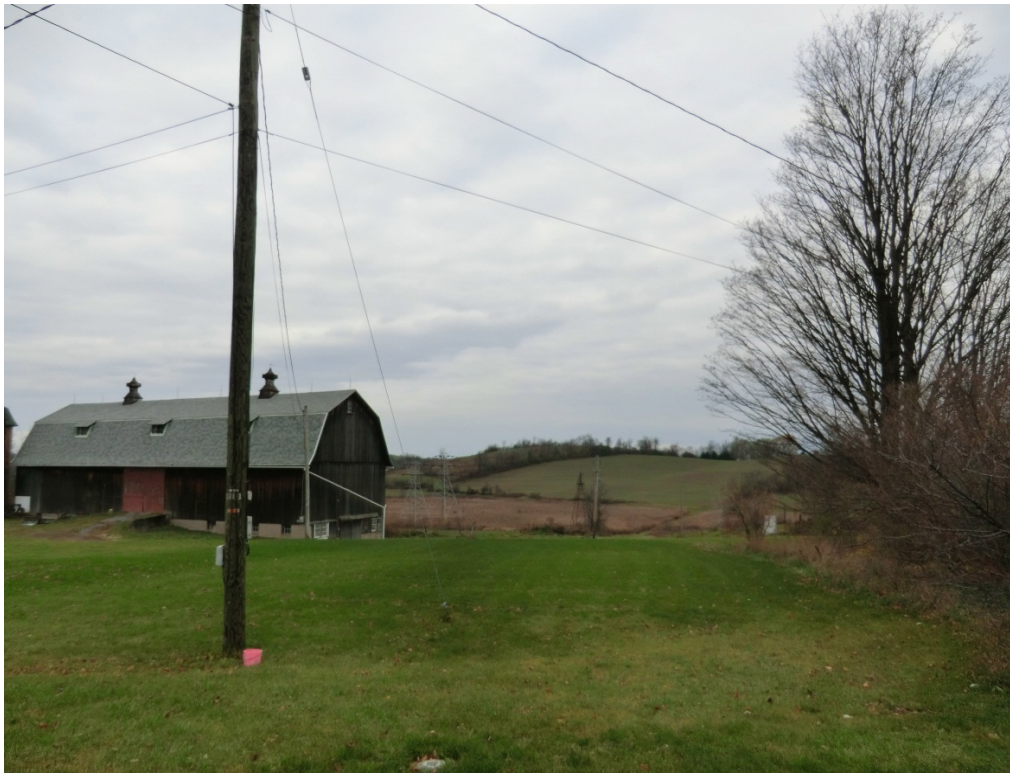
Figure 4-8 Existing National Grid ROW looking north at 8181 SR 5
