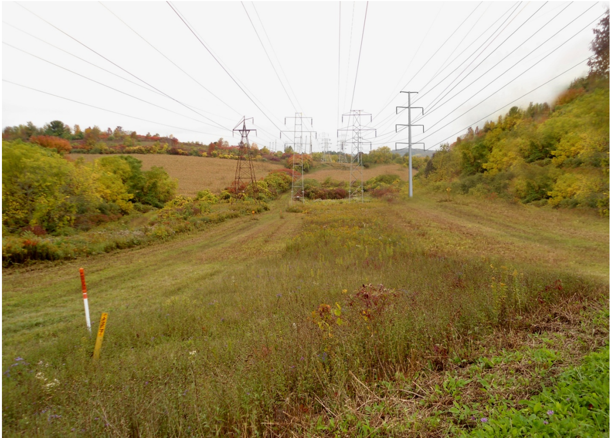
Figure 4-15 Simulation of Proposed Line on Existing National Grid ROW looking west near Kingston Road
