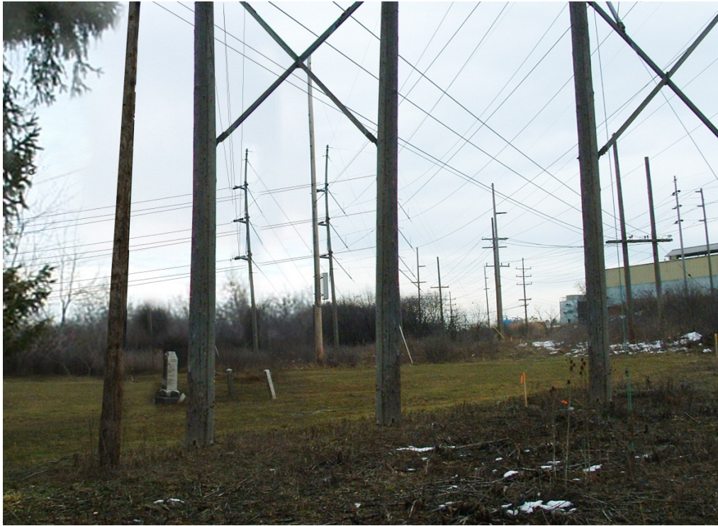
Figure 4-5 Simulation of Proposed Line on Existing NYSEG ROW looking northwest from State Street Substation toward the Cold Springs Cemetery
