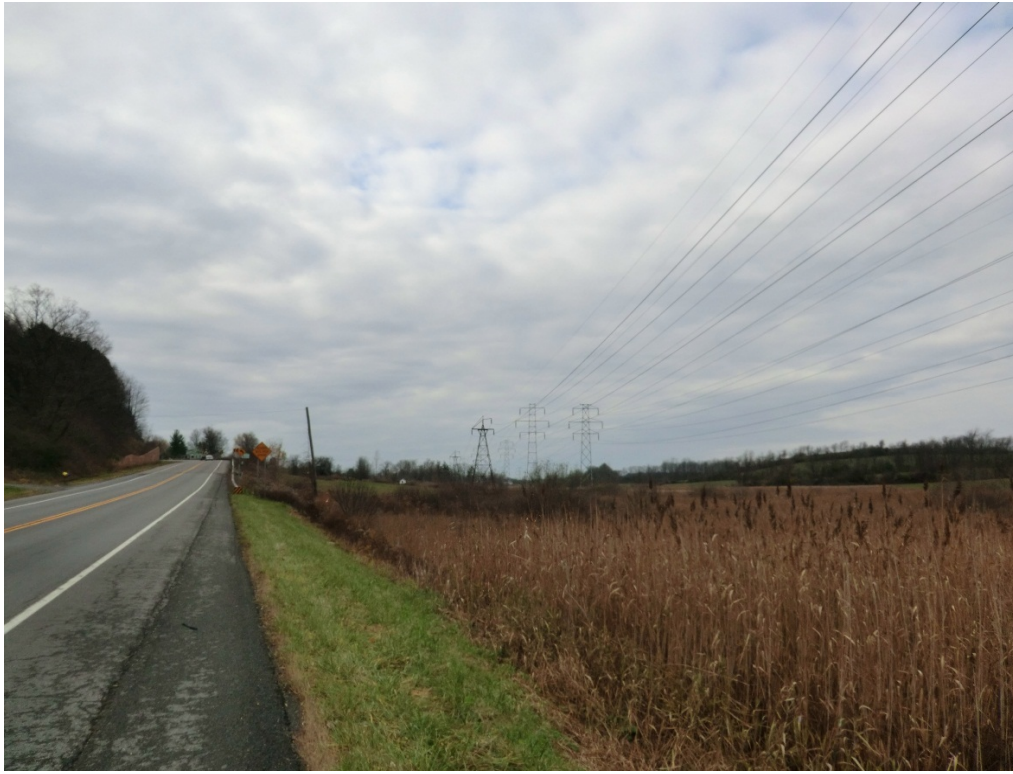
Figure 4-12 Existing National Grid ROW looking west near 8187 SR5
