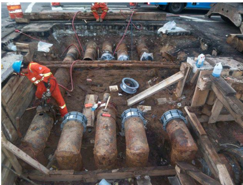
Figure 2-8. Underground Gas Manifold 12
