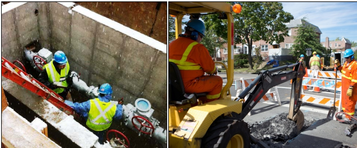
Figure 2-4: Installation of Con Edison Gas Main and Regulator Station
