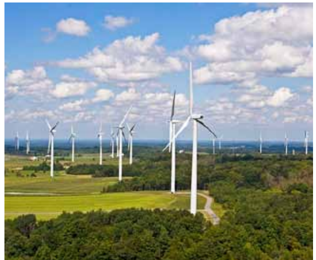
High Sheldon Wind Project
