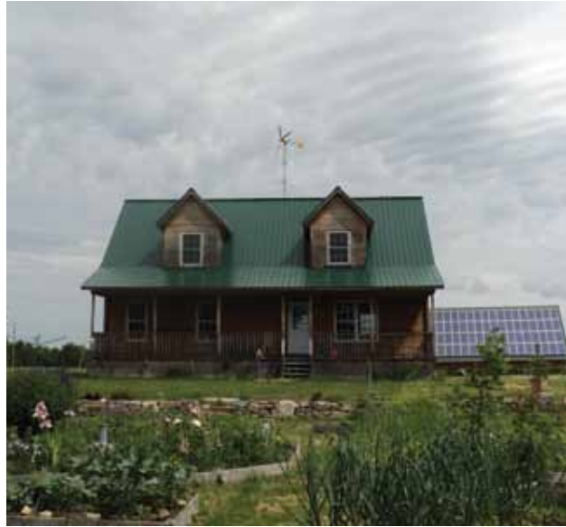
PV and On-Site Wind Systems, Ellenburg, NY.
