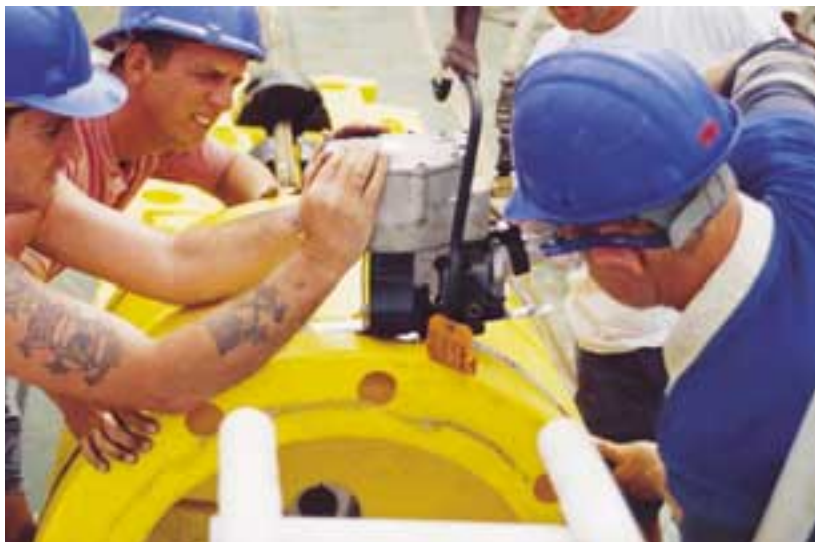
32mm pneumatic tensioning and sealing tool in operation for fast and efficient installation.
