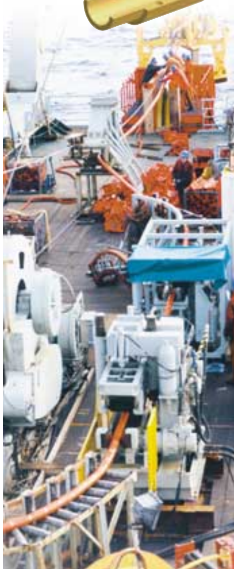
Pre-installed Uraduct® on a fibre optic cable passing through cable engines and plough
