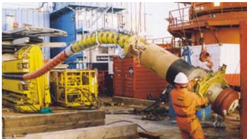
Uraduct® used in conjunction with CRP's bend restrictors on a flexible riser.
