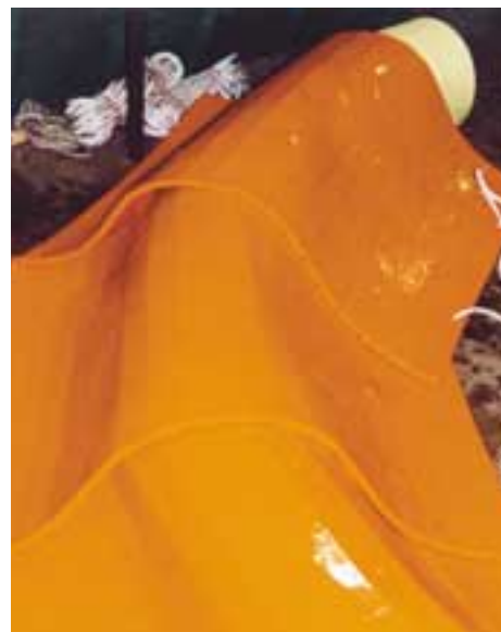
Example of Polymat deployed over pipeline.
