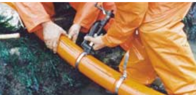
Manual hand held banding tools for diver or topside installation.
