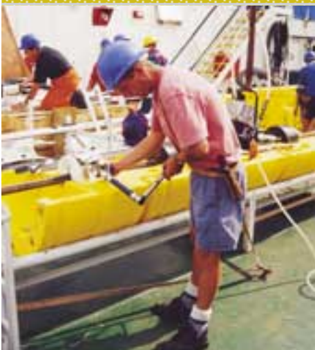
Fitting of integral cable clamps.
