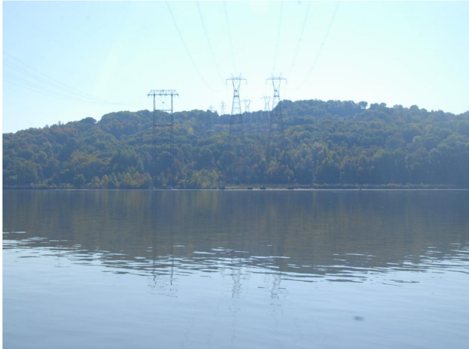
Figure 16: Existing View Easterly at Hudson River Utility Crossing, Athens NY
