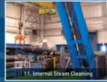
11. Internal Steam Cleaning
