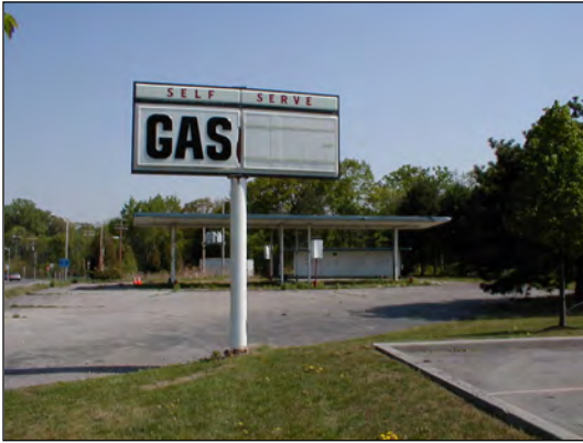
Former Payless Service Station
