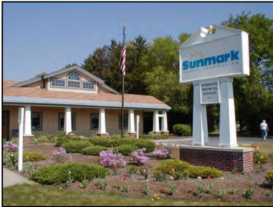
The Sunmark building exhibits the three traditional parts of a building with several roof slope planes.
