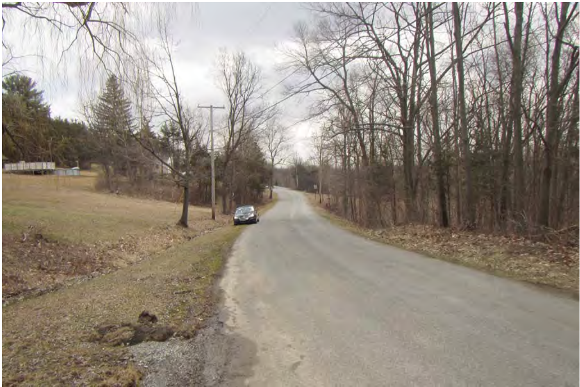
Photograph 19. Overview of conditions along Flats Extension Road. View to the south.
