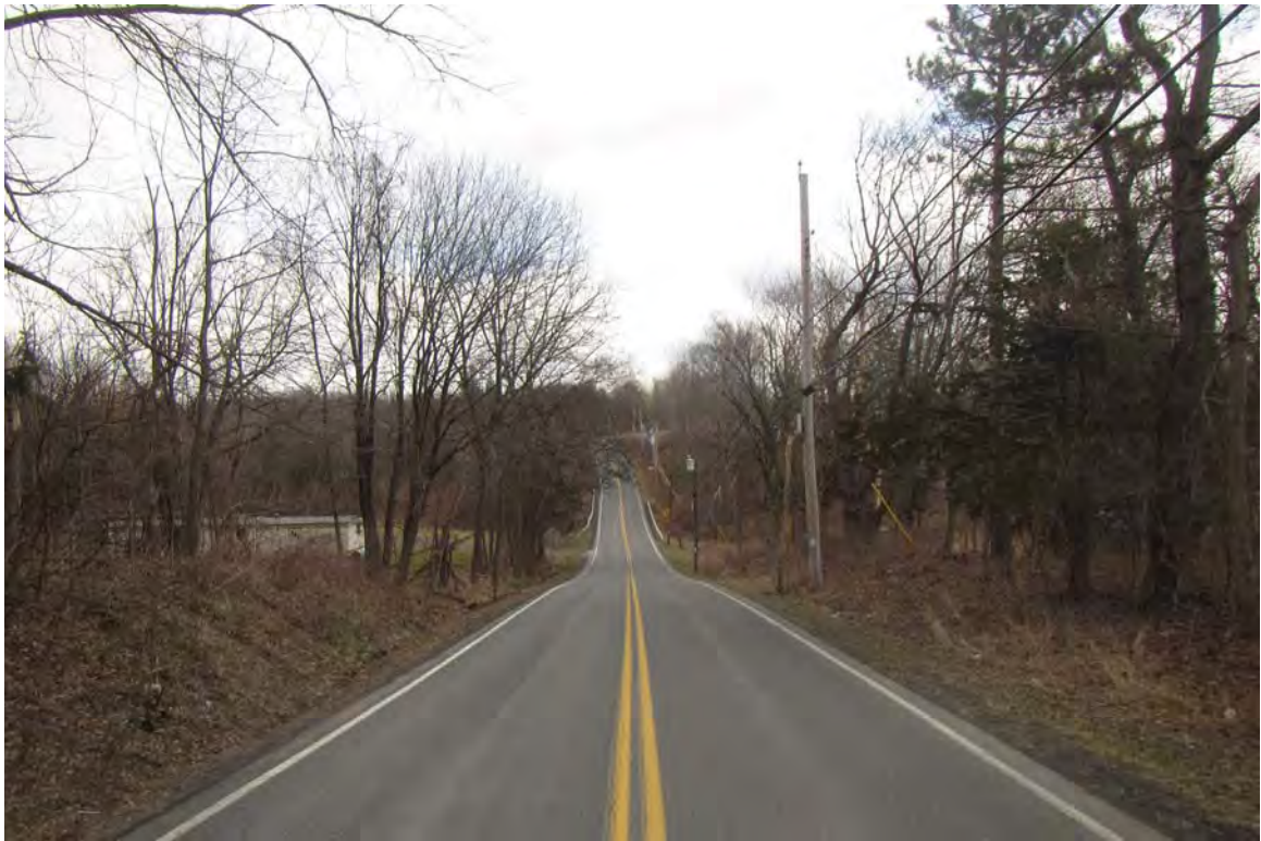
Photograph 12. Overview of conditions along Leeds-Athens Road. View to the west.
