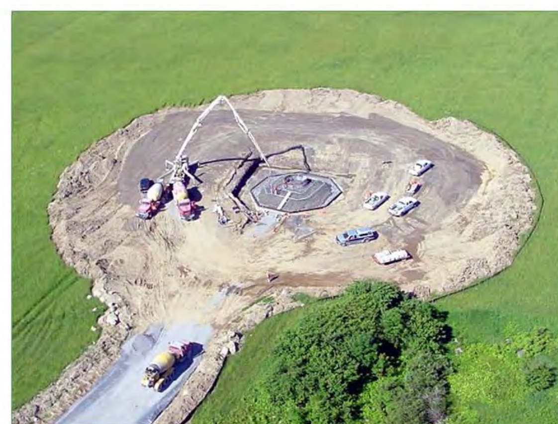
During construction, top soil gets turned back so it can be preserved.
