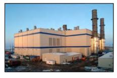
generators coupled with two heat recovery steam generators (HRSG) and a common steam turbine generator operating in combined cycle mode of operation. Key features of the project include: first GE 7FA to have black-start capability, natural gas and fuel oil fired, high level of supplemental firing and power augmentation, utilize tertiary treated water for makeup water, low emissions, enclosed steam turbine, gas turbines and HRSGs and aggressive design and construction schedule.
