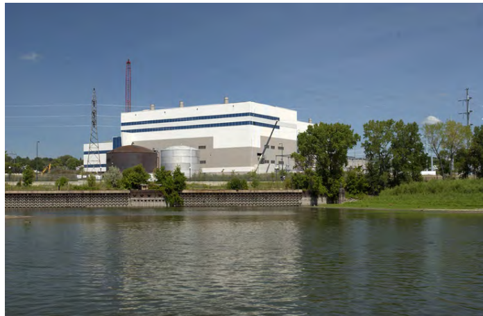
View from Mississippi river of Xcel High Bridge Plant
