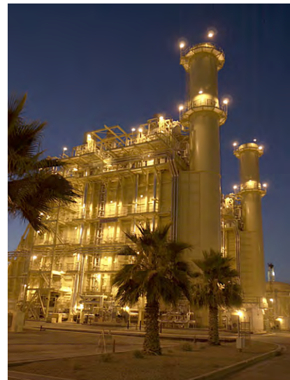
Arizona power plant at night
