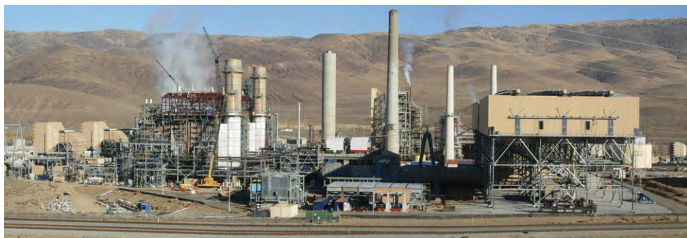
Frank A. Tracy combined cycle plant
