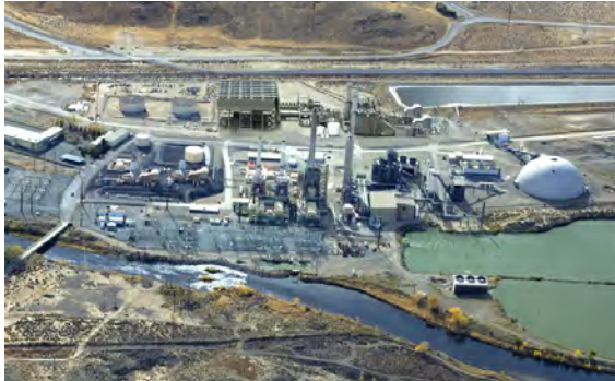
Aerial view of facility
