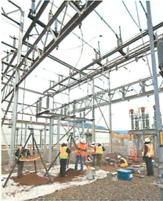
Excavation at Huth substation.
