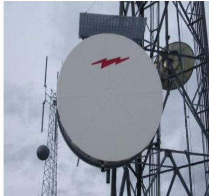
Photo 7: Tower Mounted Microwave Dish (used for backhaul typically 6 – 8 feet in diameter)
