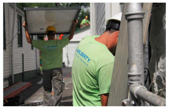
Figure 3-2: Limited space between many of the Fruit Belt Neighborhood houses prevents using a mechanical high-lift to transport the solar PV panels to the roof.
