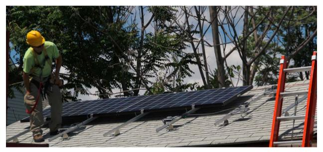
Figure 3-2: Installing solar panels at the first participant in the Fruit Belt Neighborhood Solar Project.
