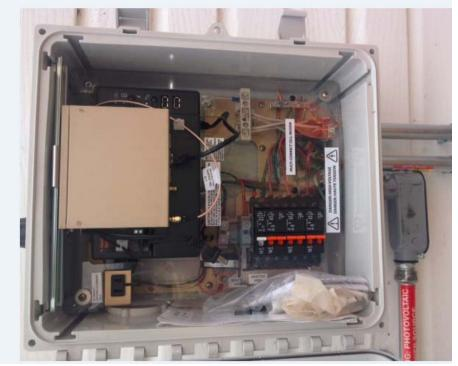
Figure 3-5: Combiner box interior where solar PV panel energy output is combined and metered before interconnection with the local electric grid.
