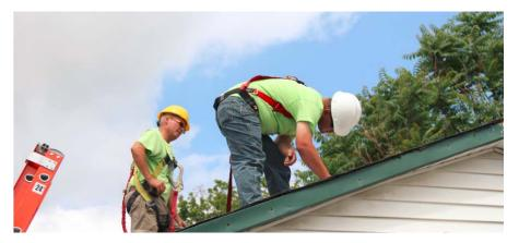
Figure 3-3: Wearing safety harnesses by all roof workers is one of several safety protocols followed by the contractor's field installation crews.
