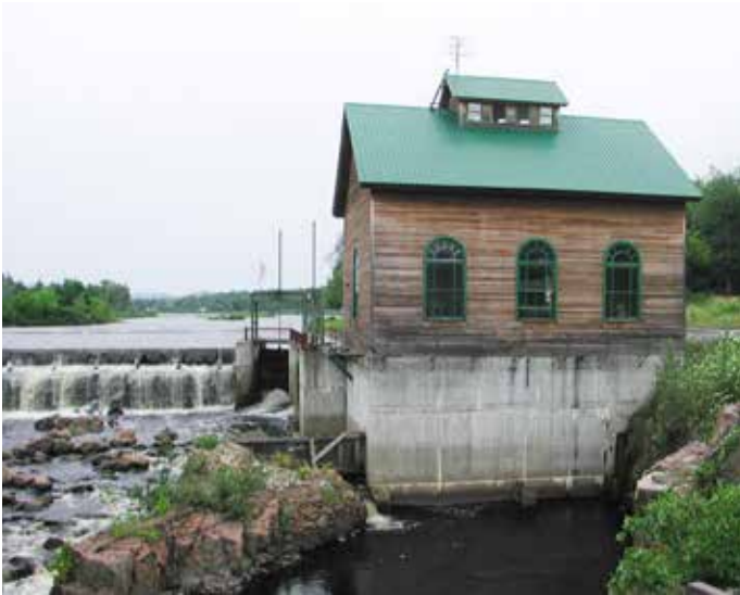
Azure Mountain Power Company, Franklin County, NY
