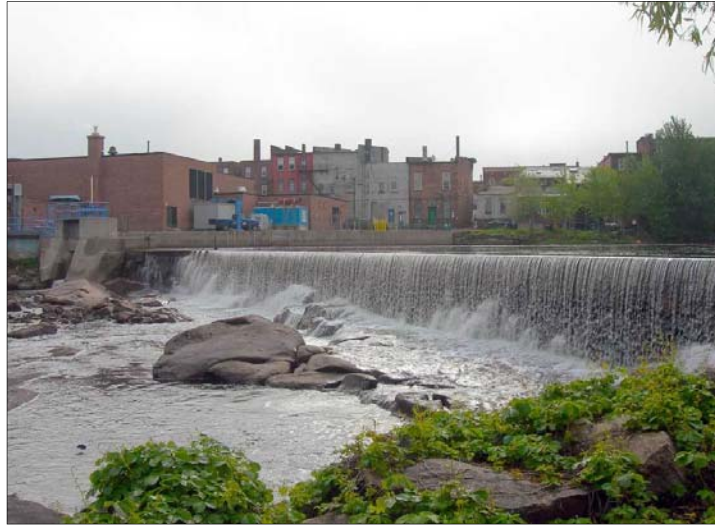
Image 2.4 – Potsdam East Hydro Facility and Dam
