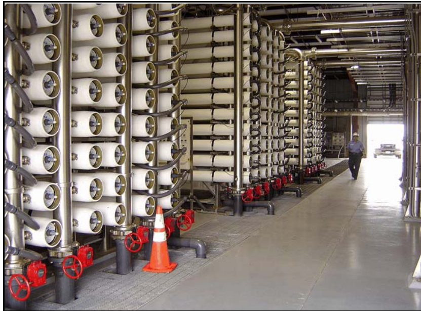
Figure 3. Three Banks of Pressure Vessels (6:11 array each) at the Southmost Facility, 2007.
