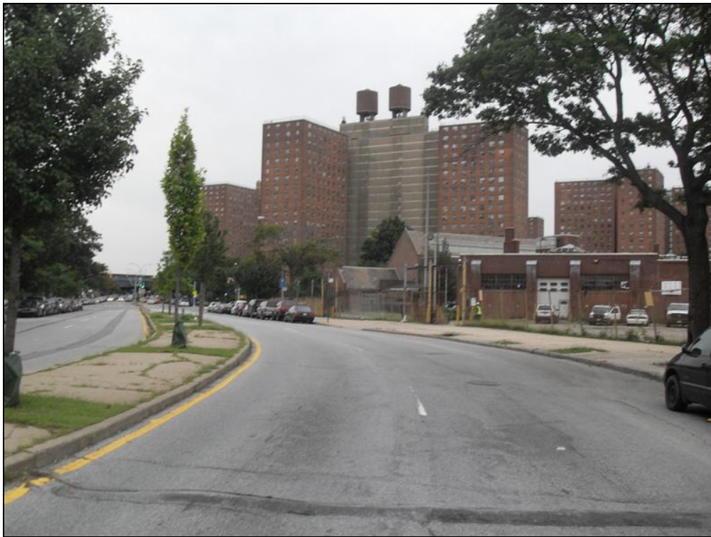
Street Scene Looking South on Shell Road (Subject at Right)
