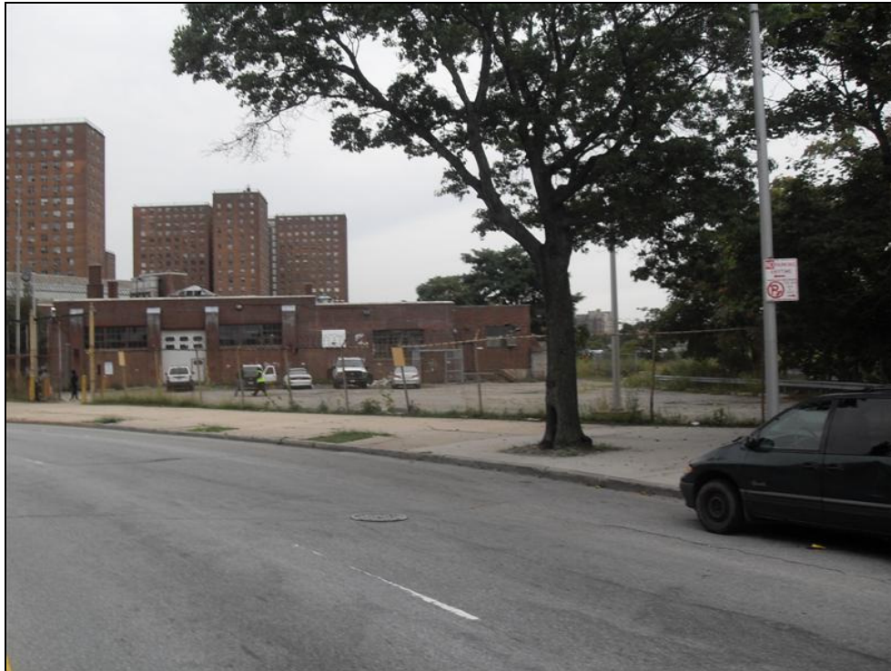
View of Subject Property from Shell Road
