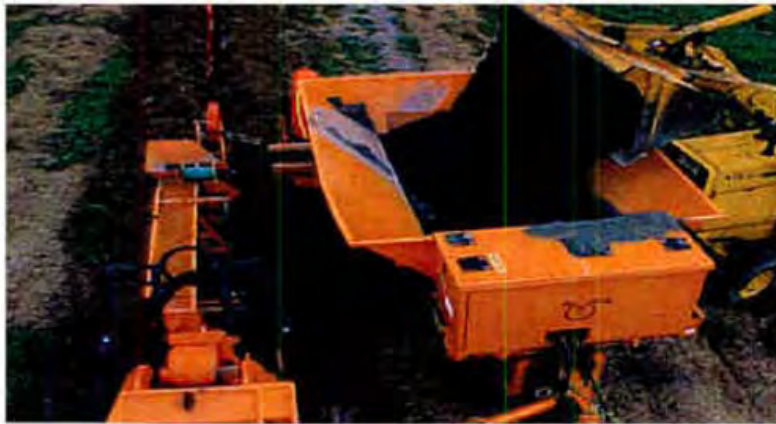
Figure 26 - Selected material placed into the can in order to be installed
