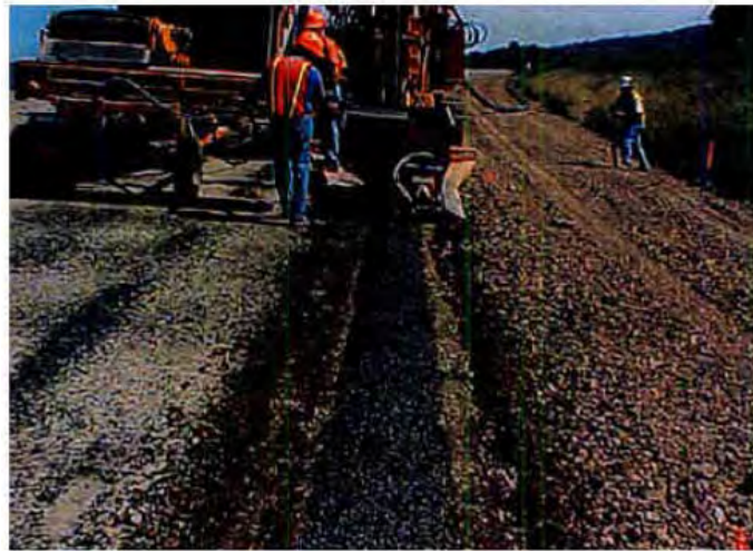
Figure 29 – Area backfilling and native soil will be placed
